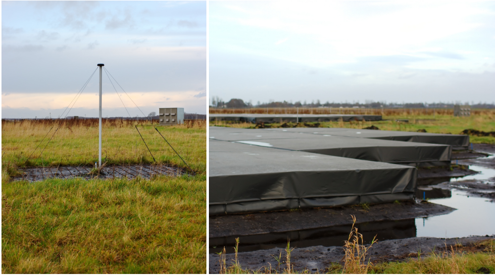
Fig. 1. Antenna types of the Low-Frequency Array. Left image: a low-band antenna with a cabin in the background. Right image: part of a high-band antenna station, consisting of 24 tiles of 4 \times 4 high-band antennas.
