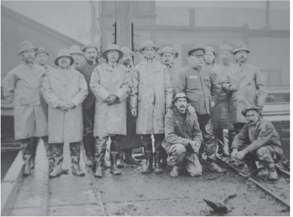
Holing through the first Hudson River Tunnel. William McAdoo ( center ), Chief Engineer Charles Jacobs ( to McAdoo's right ) and gentlemen of the press, March 12, 1904.
