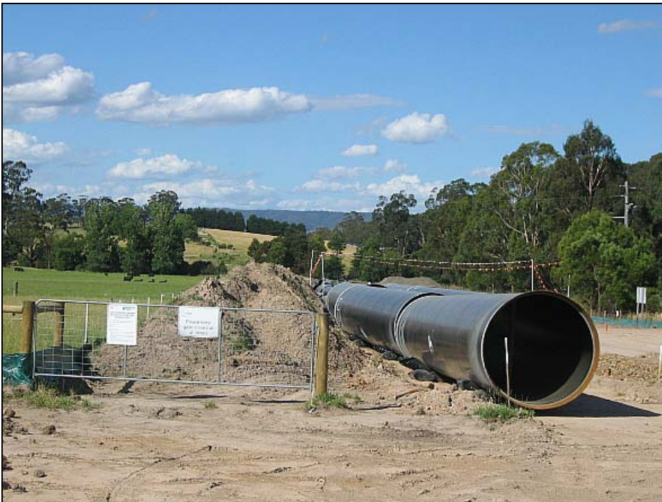
The North South Pipeline, Victoria, December 2008 (Photos: Catherine Gross)
