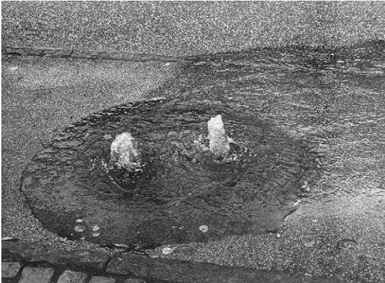
Fig. 1. Surface flooding at manhole no. 2. (Source: Jacobsen and Harremoes, 1984; reproduced with permission).
