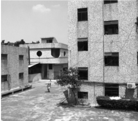
Dormitory buildings, Dongguan. Photo: Nlcnet.org
