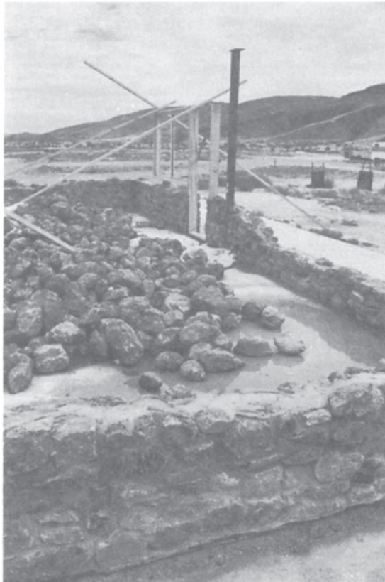
Another stone house in the making, Piplayatjarra.
