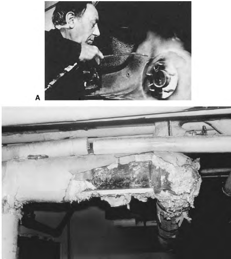
Figure 18-8. Examples of occupational exposure to asbestos: (A) Brake mechanic exposed to asbestos fibers while using compressed air to clean brake drum. (Photograph by Nick Kaufman.) (B) Exposed asbestos pipe insulation. (Photograph by Earl Dotter.)
