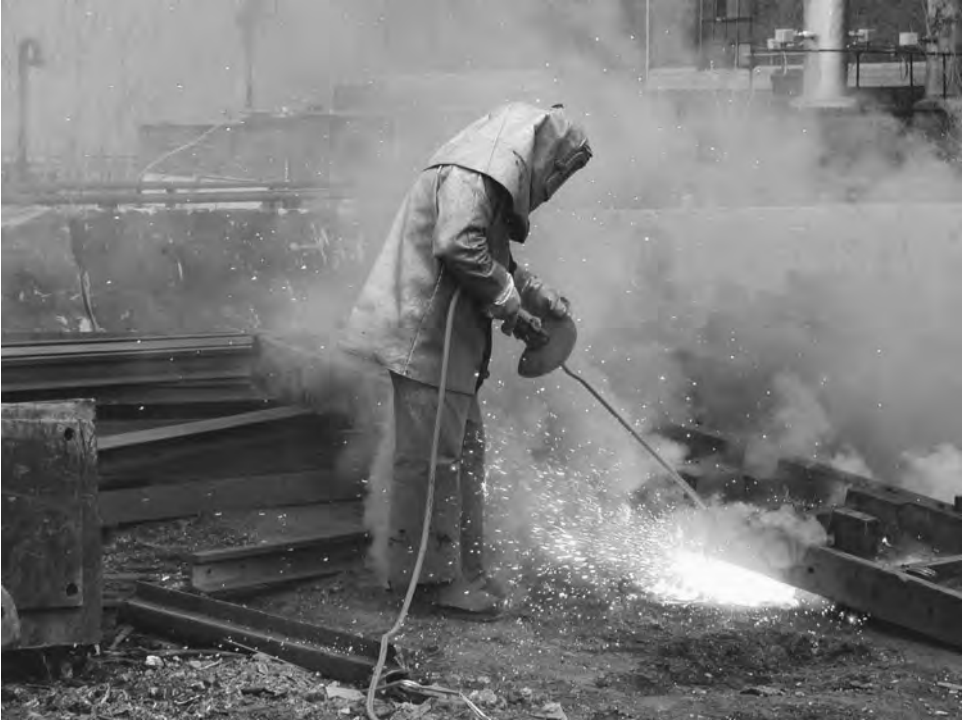
Figure 23-1. This worker is exposed to lead by cutting metal that has a lead-based coating.
