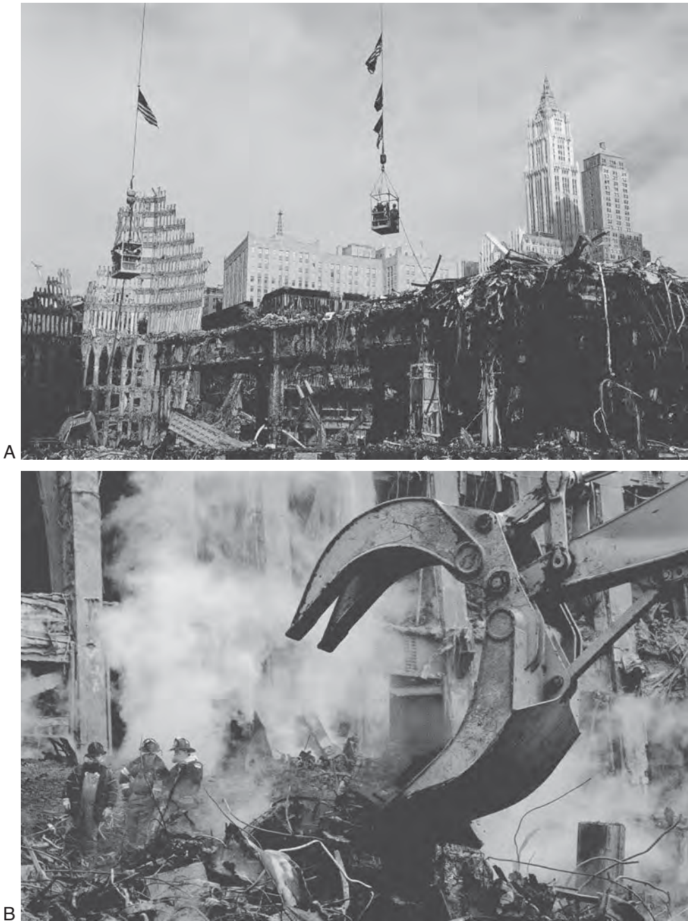
Figure 37-1. (A and B) Recovery workers at the World Trade Center site in September 2001. (Photographs by Earl Dotter.)
