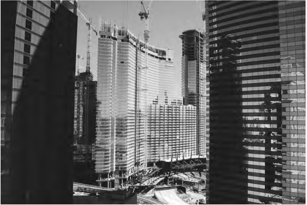
Figure 32-4. The City Center Project in Las Vegas, where the Building Trades Union negotiated for access to investigate and address the high mortality rate among construction workers. (Photograph by Barry S. Levy.)
