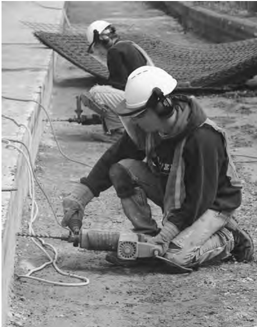
Figure 15-6. Example of worker using multiple forms of personal protective equipment, including hard hat, face shield, hearing protection, work gloves, knee pads, and work boots. (Photo courtesy of Mine Safety Appliance Company.)
