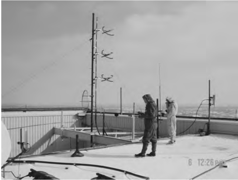
Figure 12C-6. Researchers conducting radiofrequency (RF) measurements near television broadcast antenna atop a high-rise building.
