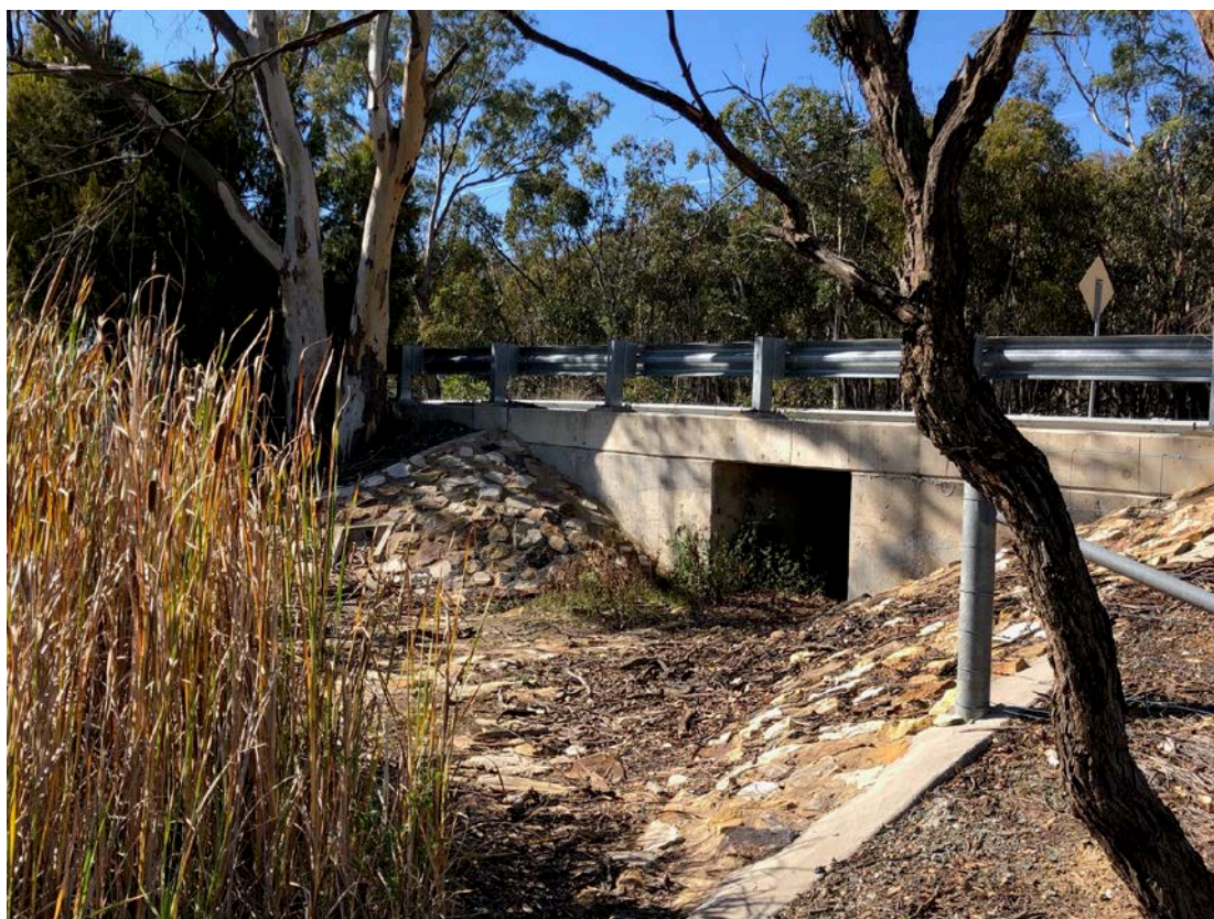
Figure 7.32 Wildlife underpass, Mulligans Flat Road
