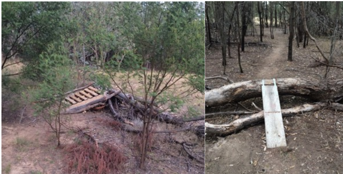
Figures 6.40 and 6.41 Construction of bike tracks and jumps
