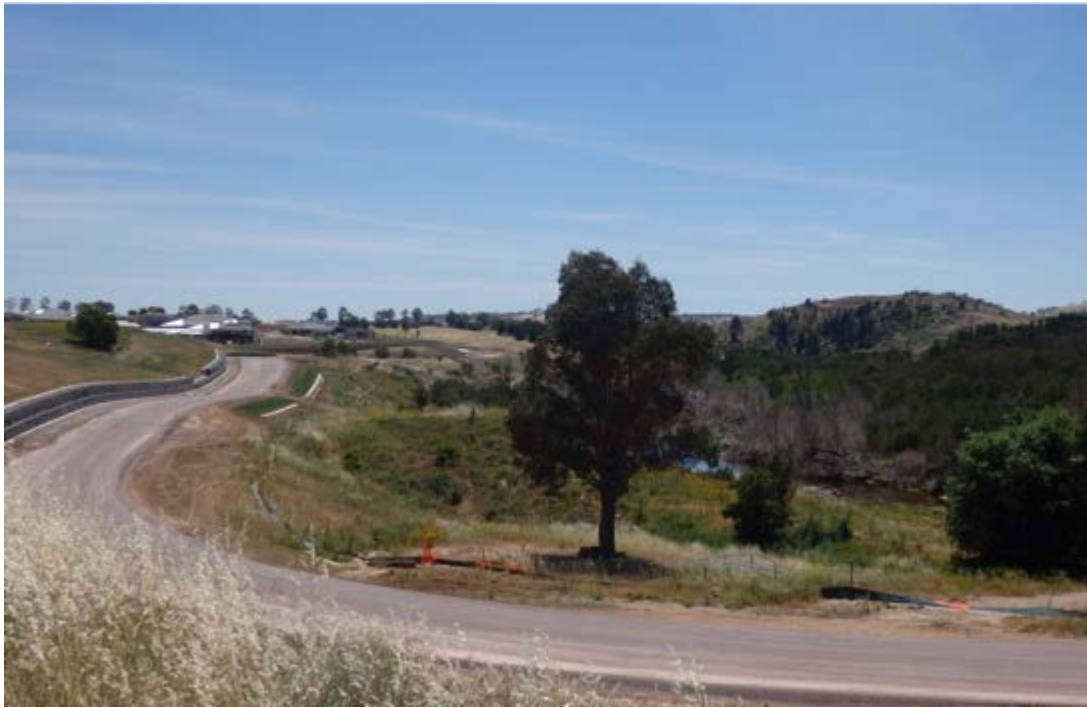
Figure 5.63 The riparian edge near Coombs (erosion control in foreground)
