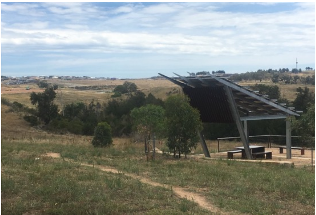
Figure 5.67 Shelter structure and trees planted for shade
