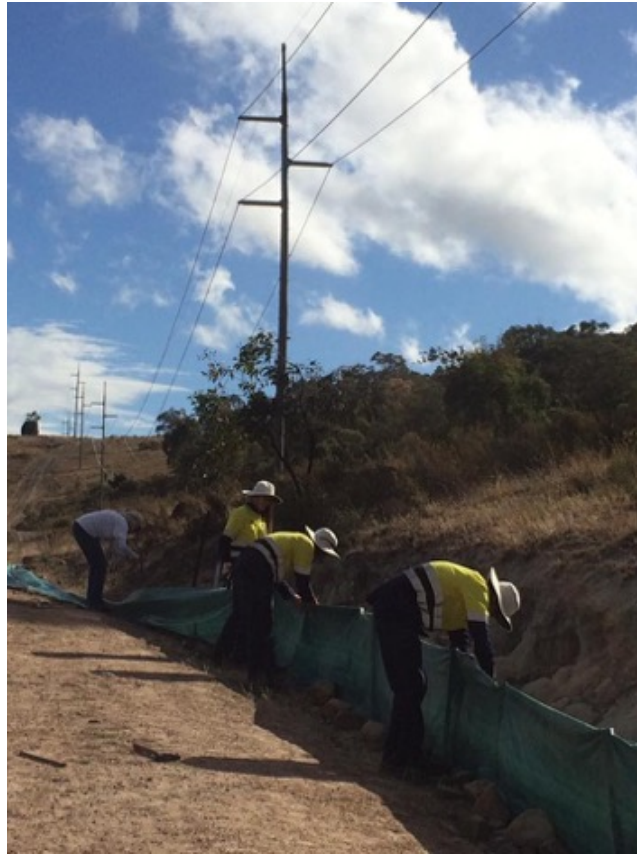
Figure 5.37 Erection of a silt fence along the western powerline trail in 2017
