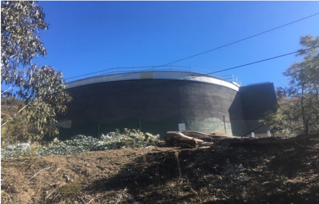
Figure 8.6 Managing utility agencies and their impacts
