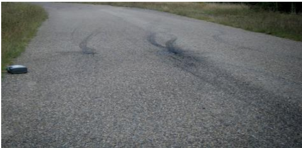
Figure 6.35 Oil and skid marks on the reserve access road
