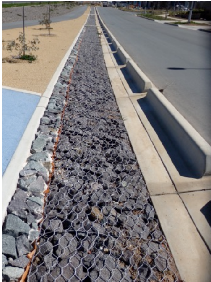
Figure 7.15 Water-sensitive drain design and tree planting in Wright
