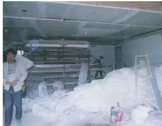
Figure 4.19 Working conditions at a hotel construction site in Kunming, 1999.
