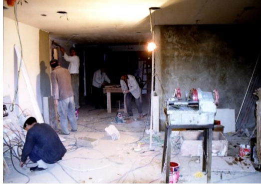
Figure 4.18 Working conditions at a hotel construction site in Kunming, 1999.
