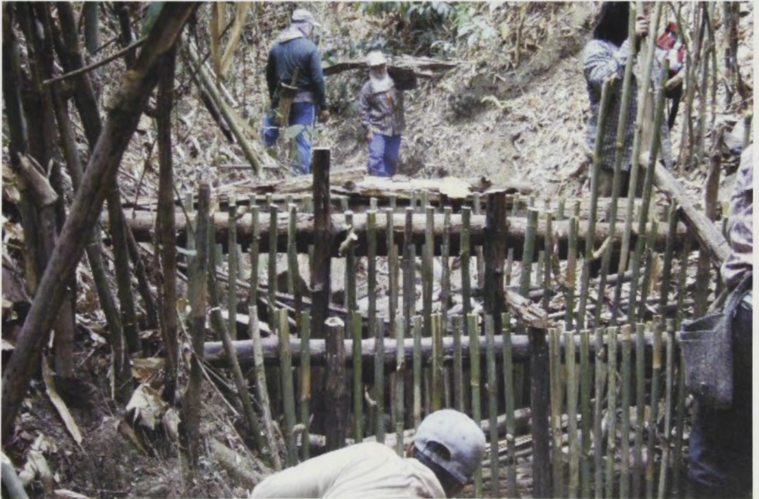
Figure 3.7 Check Dam ( Fai Maeo ) Building
