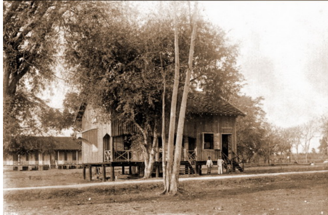
Figure 7.2: Banteay Chhmar Government Building 1924 (Collins, 2010)
