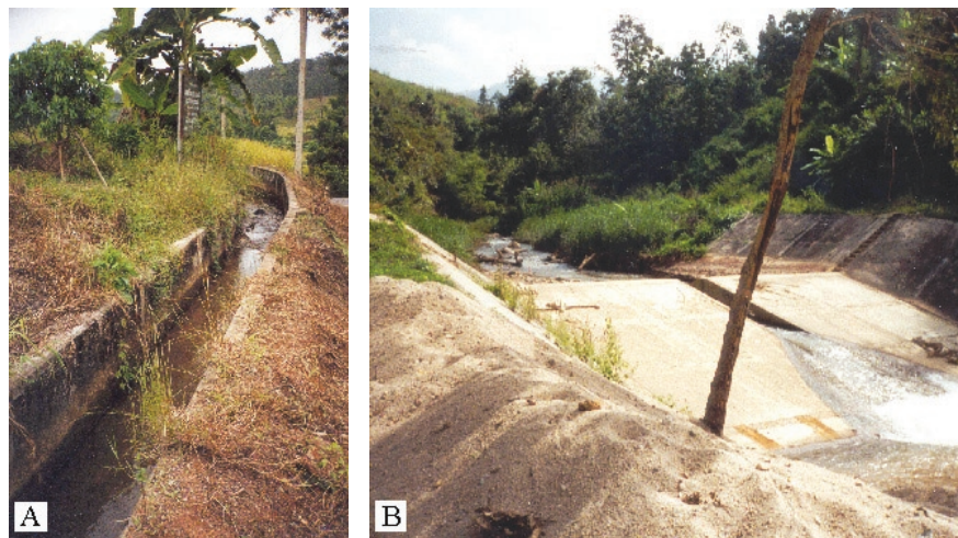
Figure 2.11 Examples of irrigation structures in sub-catchments of the Mae Chaem, northern Thailand: (A) a small irrigation canal in the Mae Pan sub-catchment; (B) a weir in the Mae Pan sub-catchment. Photos by W.S. Merritt, November 2000
