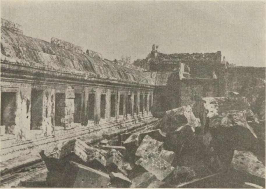
The west gallery of the sanctuary enclosure. The pile of stone blocks in the foreground represents what is left of the sanctuary tower
