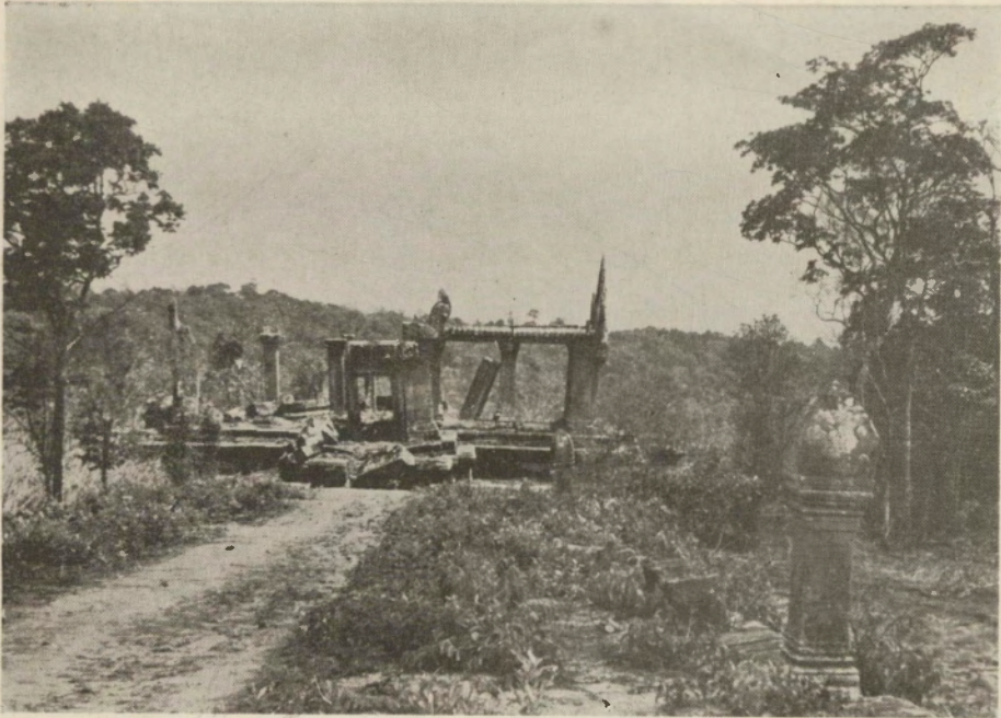
The first gopura viewed from the south, with one of the menhir-like border markers of the first causeway at the right.
