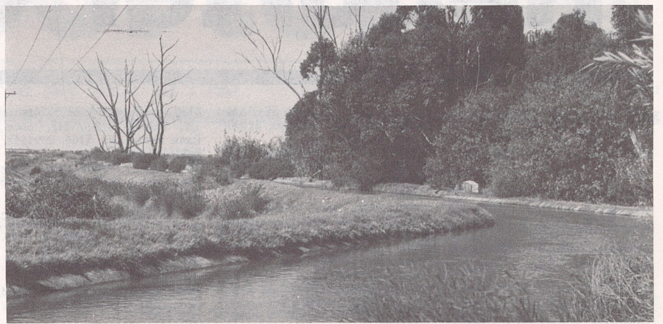
Irrigation channel in the Mildura area
