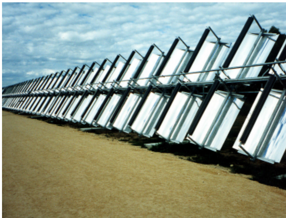
Figure 1-1: 20kW PV/Trough demonstration system at Rockingham, Western Australia. The array is ~100m long.
