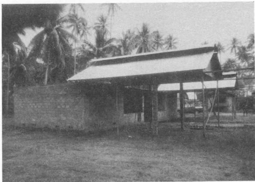
Plate 5 Ceylon drier with sliding roof, producing hot-air quality copra
