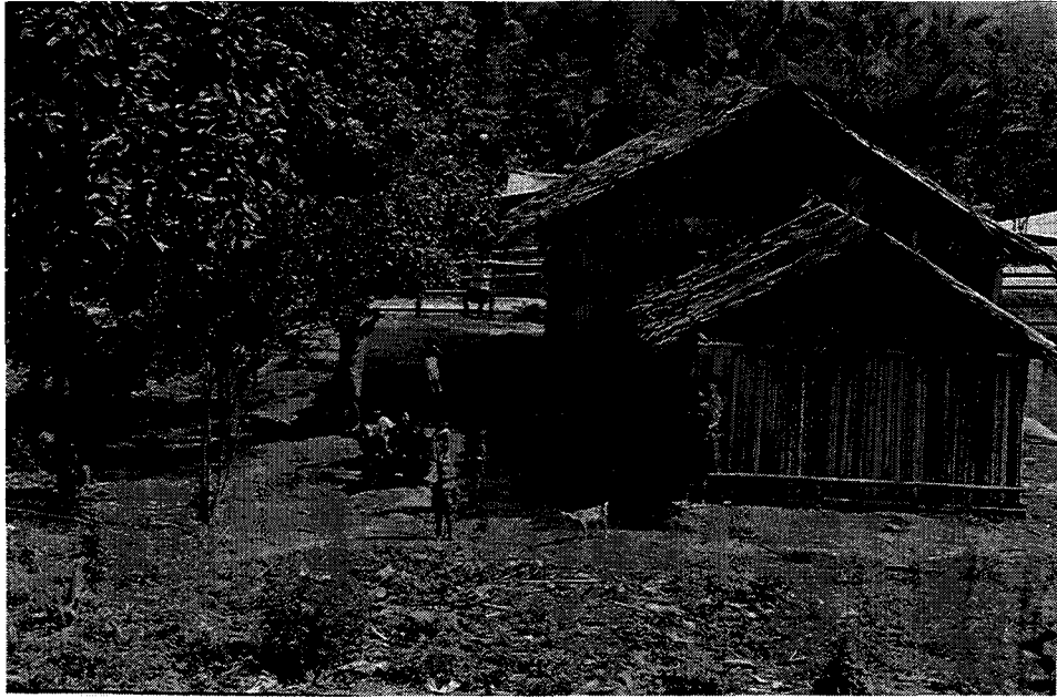
25 Village house and its rear kitchen
