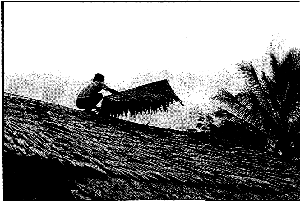
27 Putting a female thatch on the ridge of the roof
