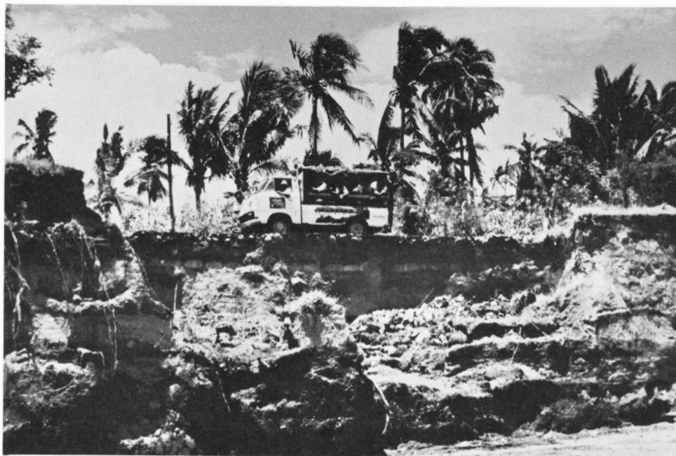
Plate 28 River Nanga Limang, 2 km south of Maumere; heavily damaged embankment caused by annual floods, whereby main road ( Floresweg ) between Nita and Maumere was partly washed away.
