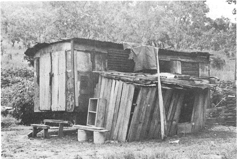
Plate 17. Converted caravan with lean-to kitchen.
