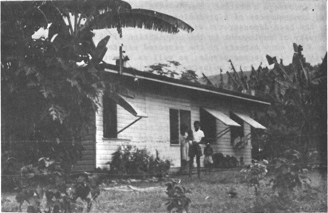
Plate 3. Earliest design weatherboard house 'without amenities'.
