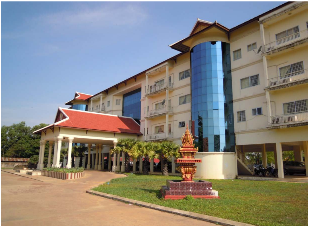
Figure 12. Preah Vihear Provincial Municipality building. (Photo by the author.)
