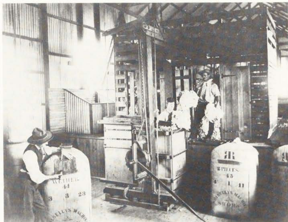
39 Manually operated wool press superseded the lever type, which required a strong operator
