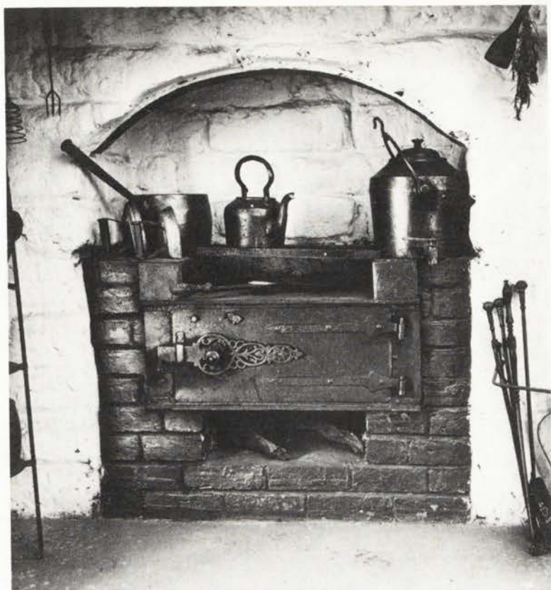
A colonial or two-fire stove; an early fuel stove which was soon replaced by a stove with a single firebox. By courtesy of Swan Hill Pioneer Settlement.
