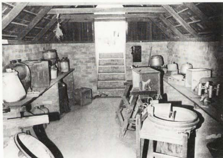
A half-cellar, built partly underground for coolness. Widely overhanging roof and slope of the ground prevent rain from entering. By courtesy of Swan Hill Pioneer Settlement.
