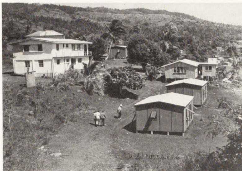
Plate 4 Substandard housing in urban area
