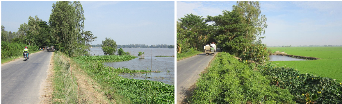
Figure 4.6 An embankment dyke of North Vam Nao project in Phu Xuan with the flood season (left) and the winter-spring crop after flood recession (right)
