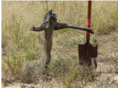
Figure 5-3. Exposed lateral roots of an old tree stump showing extent of soil loss.
