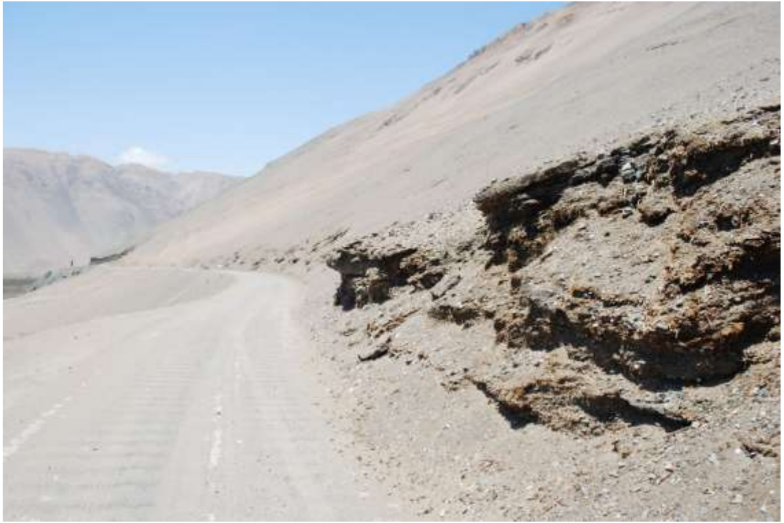
Figure 4.2: Exposed midden- Caleta Camarones. This deposit was cut by road construction. Note the presence of vegetal material along with shell and bone. Photo: C. Carter
