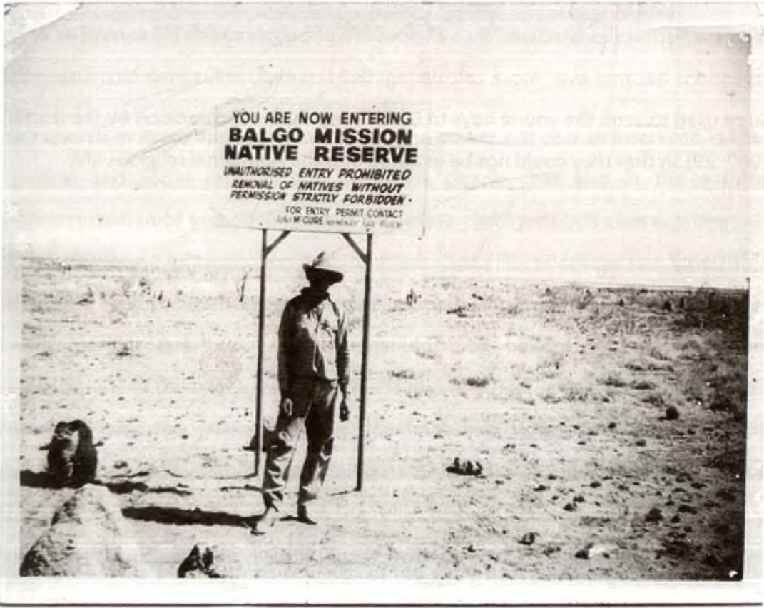
Figure 1.3. Stockman George Tuckerbox under a sign erected by Father McGuire at the entry to the new Balgo Mission, mid 1960s. (Photo by Joe Mahood, © Kim Mahood)
