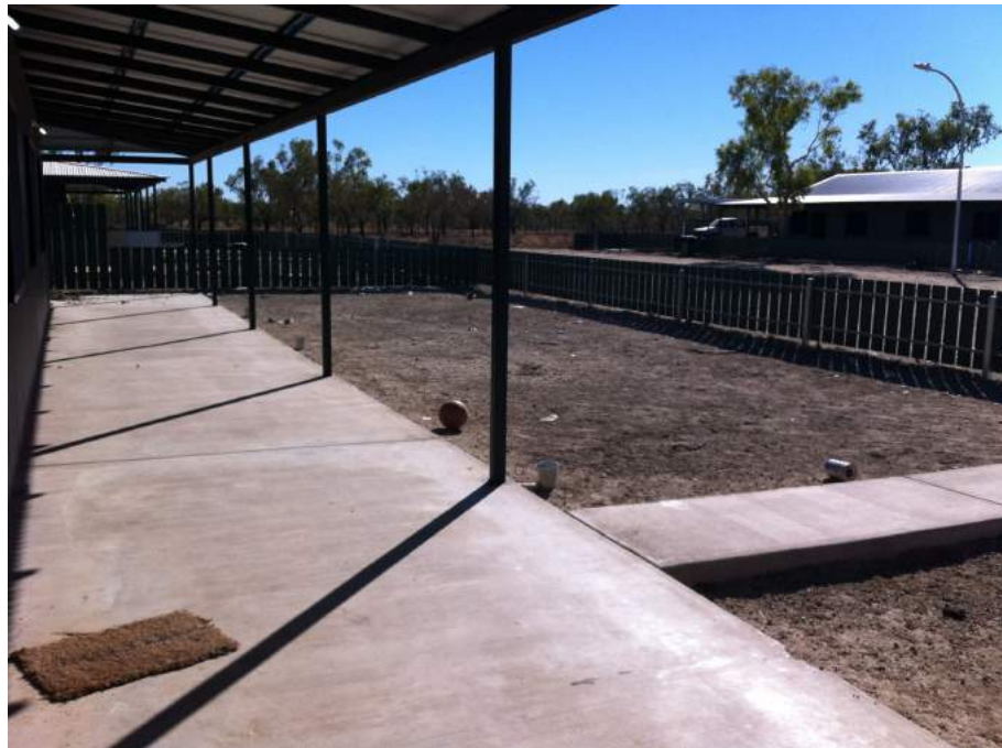
Plate 2.16 New housing at Warrmarn , 1 st August 2012.
